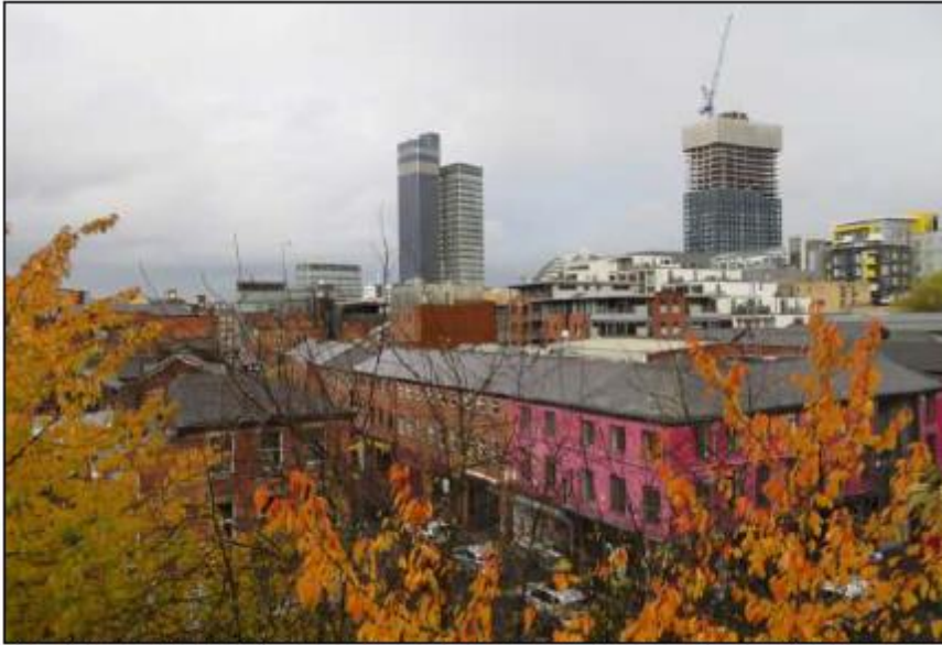
Fig 8. View across Thomas Street from the roof of the car-park (November 2018) showing the variety of the roofscape across the conservation area and the uniformity on the north side of the street.
